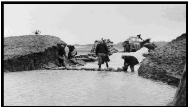
Wells-next-the-Sea, repairing sea wall, 1953. Source: picture.norfolk.gov.uk
